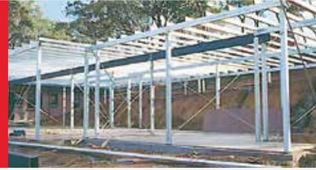
Wind pressure produces horizontal loads on the DuraGal Flooring System. For free standing floors these loads are transferred to the footings through the use of sub-floor bracing.
