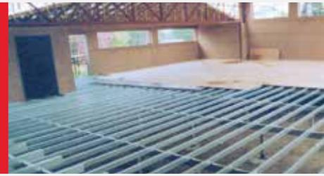
Whether the DuraGal Flooring System is used in brick veneer or free standing construction, assembly is straight forward and uncomplicated. The following is a typical step by step procedure.
