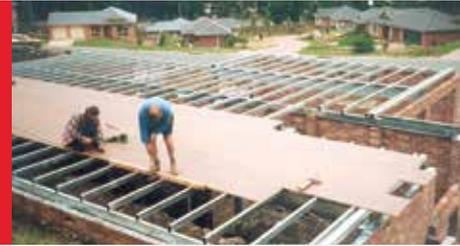
For brick veneer construction, there are many ways of fixing the DuraGal Flooring System to the brick work. The method used depends on the wind category and building preferences.
